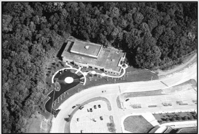
An aerial view of the Setzer Pavilion/Mills Morgan Center
